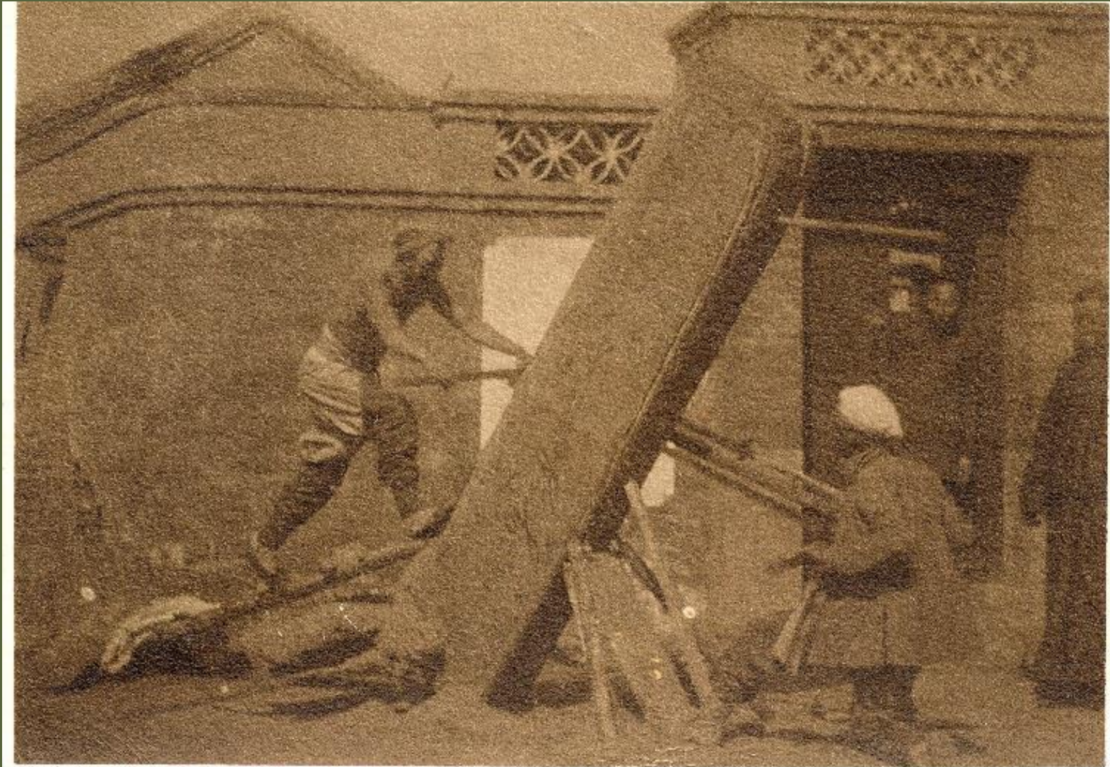
Sawing wood into planks
